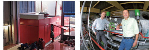
Installation of the CHP system Engineers at the Trier Factory, Germany
