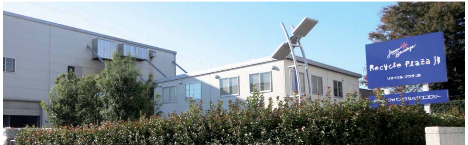
The Recycle Plaza JB disposal facility
